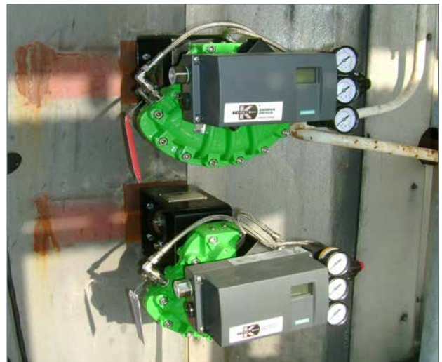
TYPE K DM Series on Windbox application
