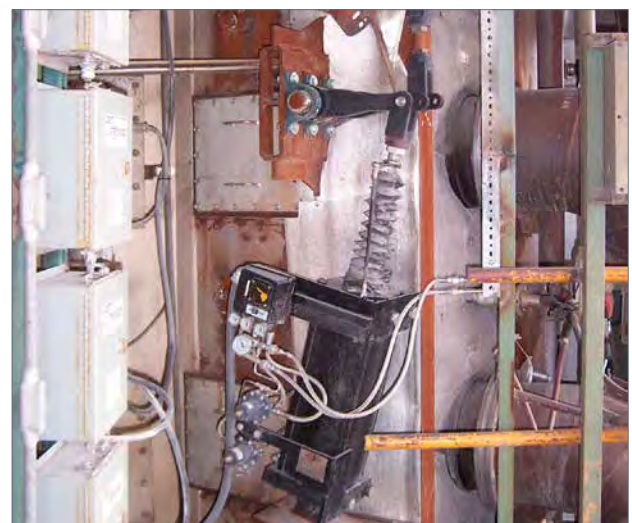
Burner Nozzle Tilt Drive
