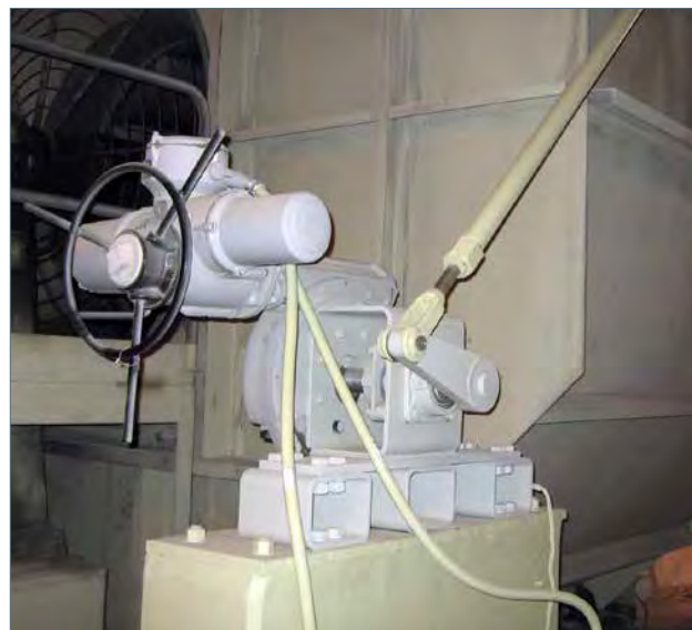
IQ Series on ID Fan Inlet Damper
