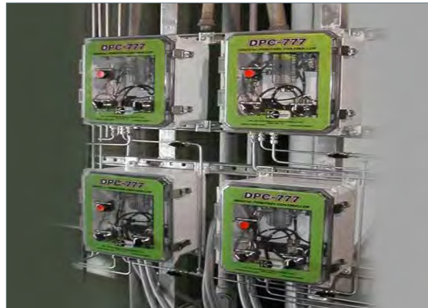
Remote Mount Digital Position Controller
